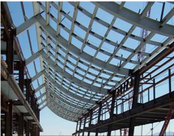
Norman Y. Mineta Airport Construction
